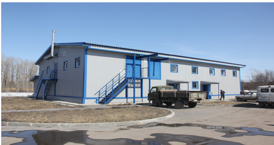
Figure 3. Building of the sewage treatment plant in the workers' settlement of Maslyanino, Novosibirsk Region
